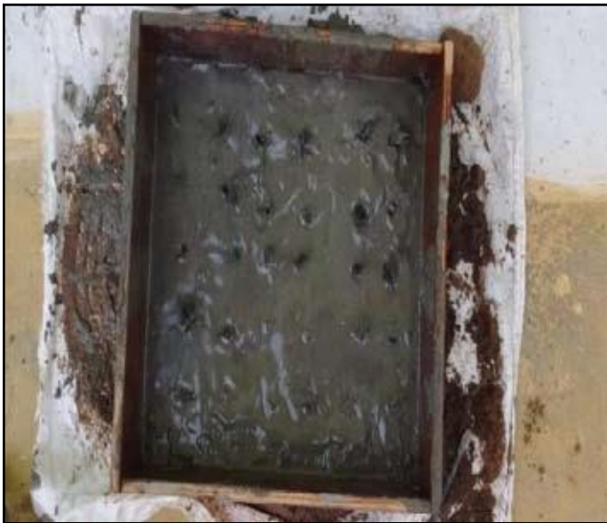
Fig 6: Pouring of concrete in mould
