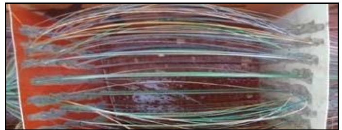
Fig 4: fixing of fibre
